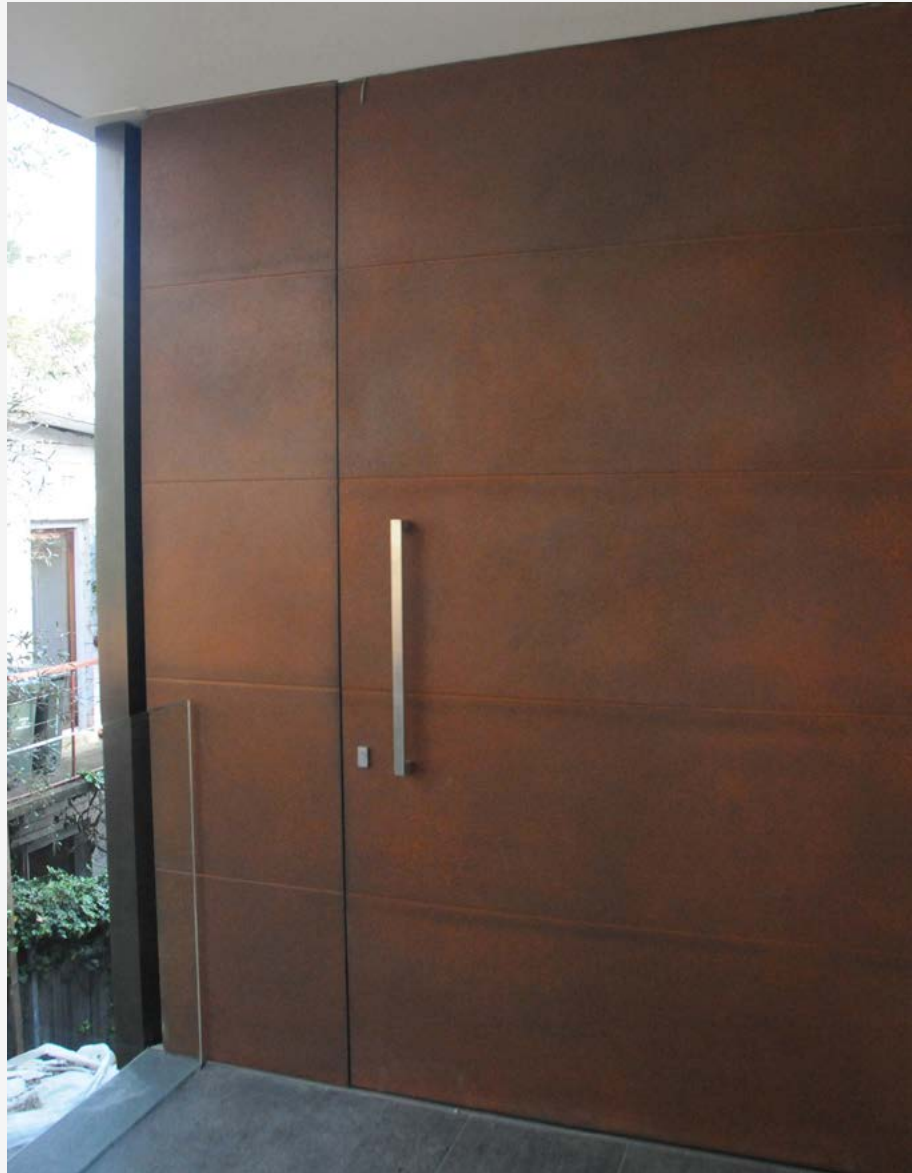
Brown Rust | Channel Door
